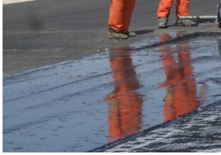
Figure 1: Finely milled substrate Figure 2: Mirror effect of fresh bond coat/black prints on product
