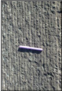
Figure 1: Finely milled substrate Figure 2: Mirror effect of fresh bond coat/black prints on product
