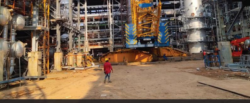
The working platform for the crane lifting refinery components had to support a maximum load of 23t/m2, with a maximum allowable settlement of 75mm
