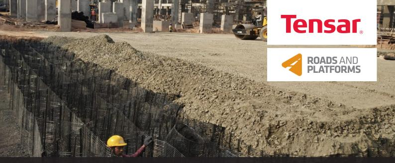
Both platforms comprised a 1m thick mechanically stabilised granular layer (MSL), with additional bearing capacity in the lifting area provided by a 0.65m thick TensarTech Stratum basal mattress below the 1m MSL.
